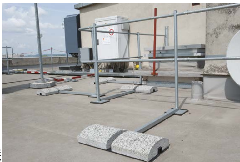
Photo 8. Garde-corps autoportant
